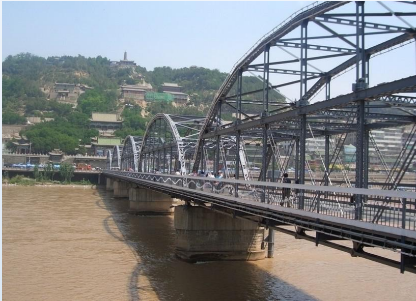
The Lanzhou Zhongshan Bridge
